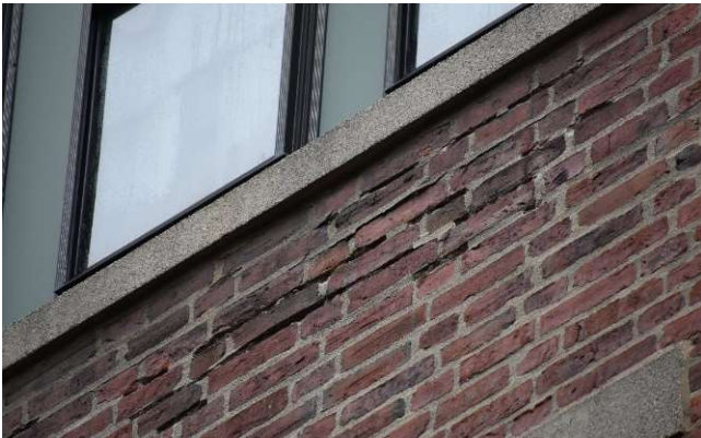
Deteriorated Mortar
