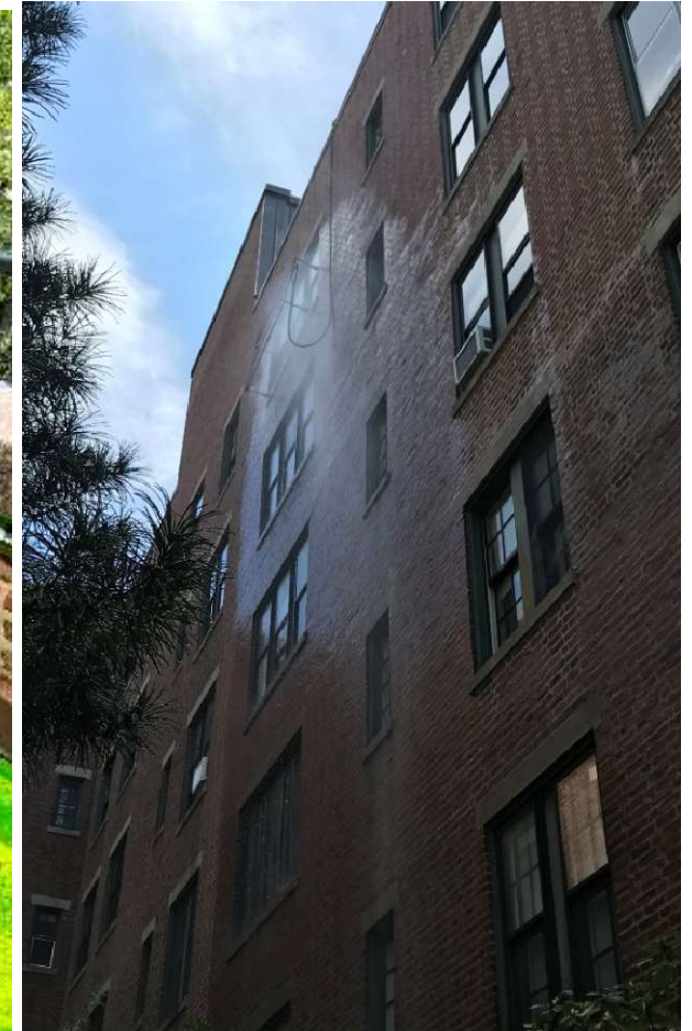
Spray Rack Testing
