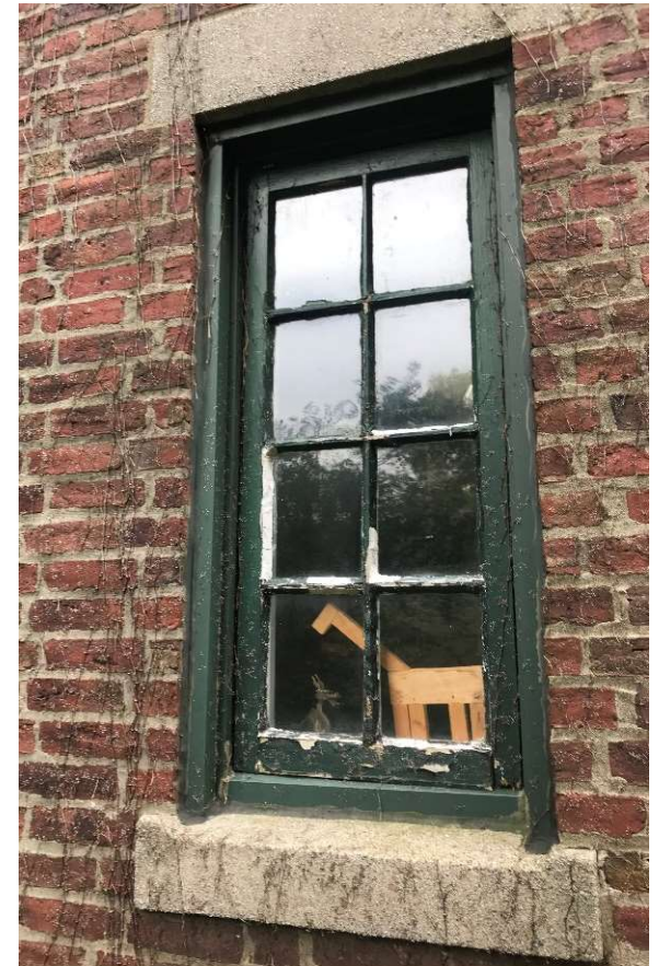
Deteriorated Window
